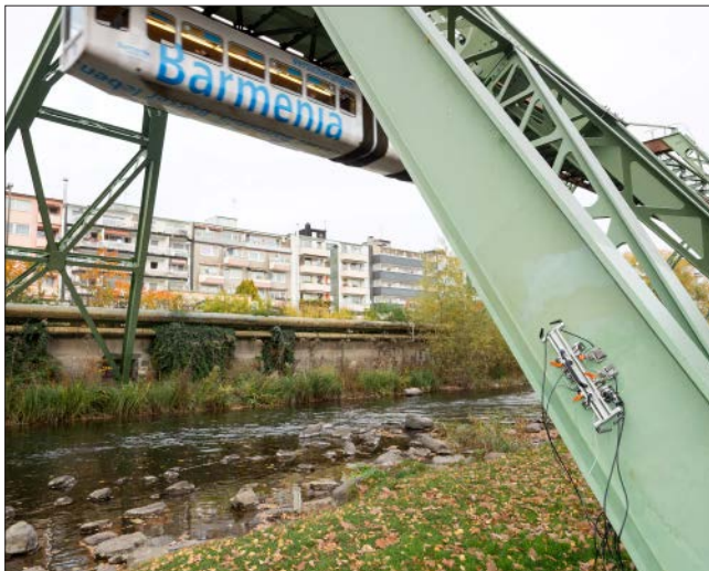
Weld testing on a pillar of the famous Wuppertal Suspension Railway ...
